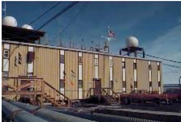
**Figure 8. The weather instrumentation shown here atop Building 165, McMurdo Operations and McMurdo Weather Office is the source of McMurdo Station's synoptic observations.**
